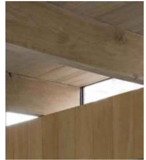
Materials and detailing
